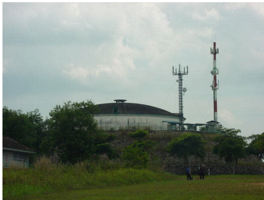
Figure 4. Photograph of Mobile Telephone Base Station Tower at Taman Daya a) left picture shows Celcom tower and b) right picture shows sharing DiGi and Maxis tower
